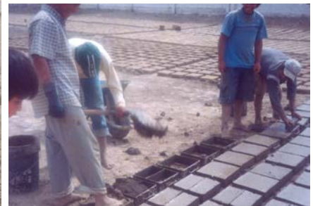
Figure 29: Adobe units under construction
