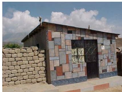
Figure 11: Adobe house facade with colorful tiles in Machaguay
