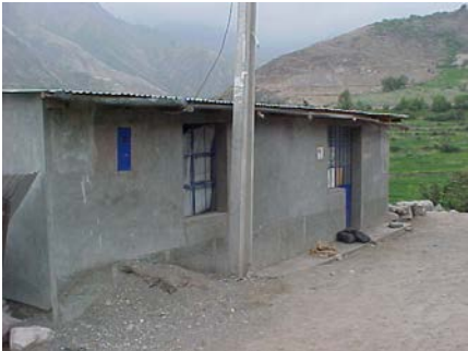
Figure 4: Windows and door centered in the walls
