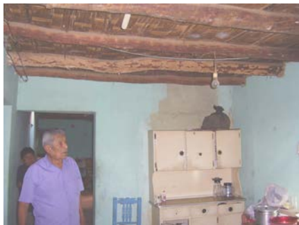
Figure 22: House reinforced in 1998 in Ica; after the 2007 earthquake. Owner Mr. Legua receives visitors showing undamaged adobe walls.
