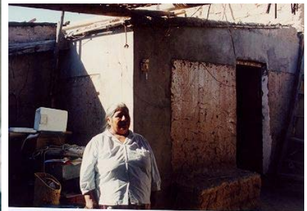
Fig. 18: Adobe house reinforced with strips of wire mesh, undamaged after 2001 earthquake in Moquegua.
