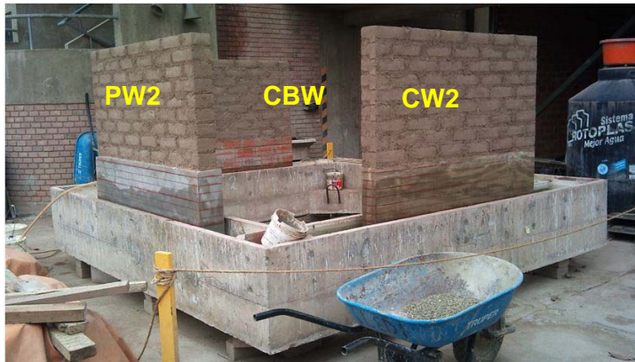
Figure 11: Three walls of set 2 that resisted the flooding simulation test
