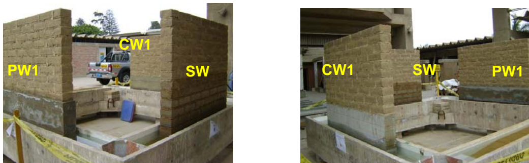
Figure 10: Three walls of set 1 that resisted the flooding simulation test
