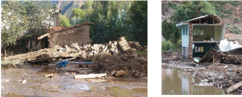
Figure1: Collapse of adobe houses under floods, Cusco Perú - 2010.
