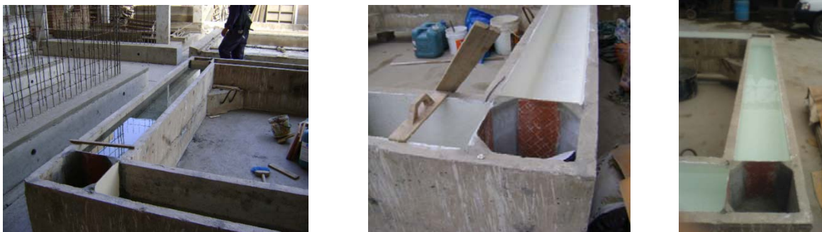
Figure 2: Channel used in the test of flooding. Test of water tightness.
