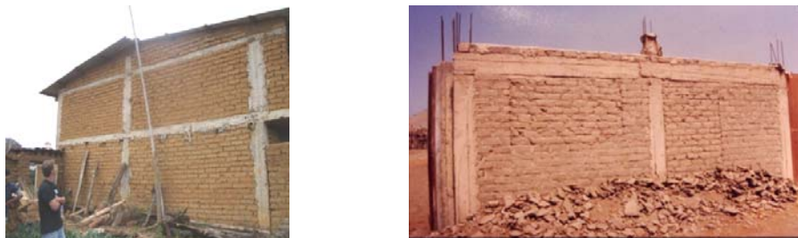
Figure 1: Examples of confined adobe walls in Peru.
