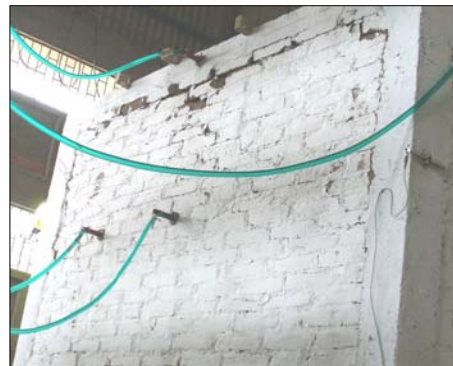
Figure 8: Second story flexure wall after step 2.
