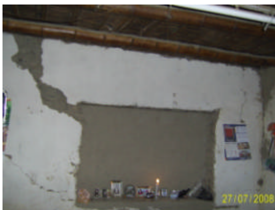
Figure 15. Non reinforced back room of the house in La Tinguiña had cracks.
