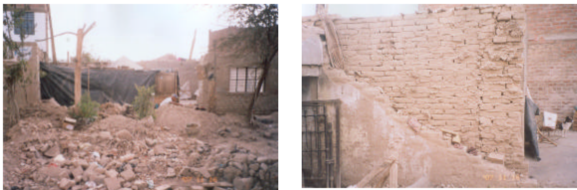
Figure 13. Demolished adobe walls in neighbor houses in Parcona
