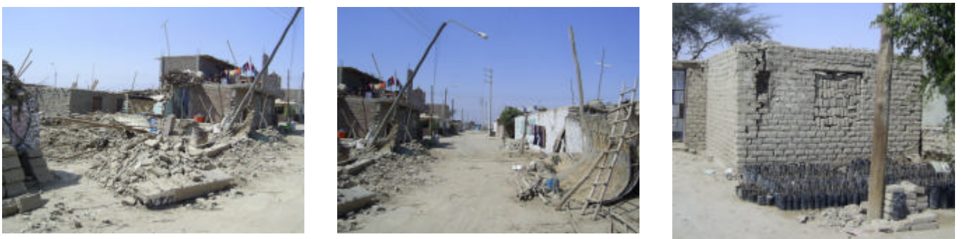
Figure 11. Traditional adobe houses with damage in Pachacutec
