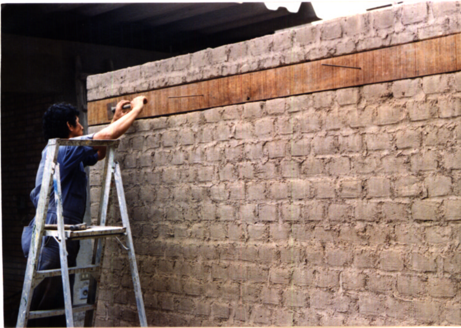
Fig. 8 Type 1 Reinforcement
