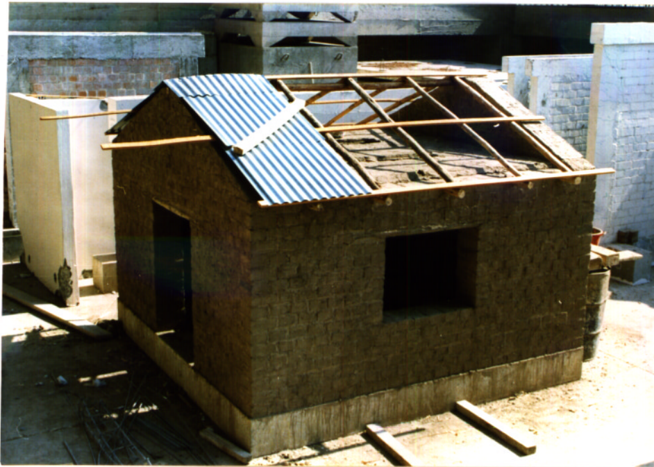
Fig. 14 Unreinforced adobe house specimen (typical of the Andes) under construction
