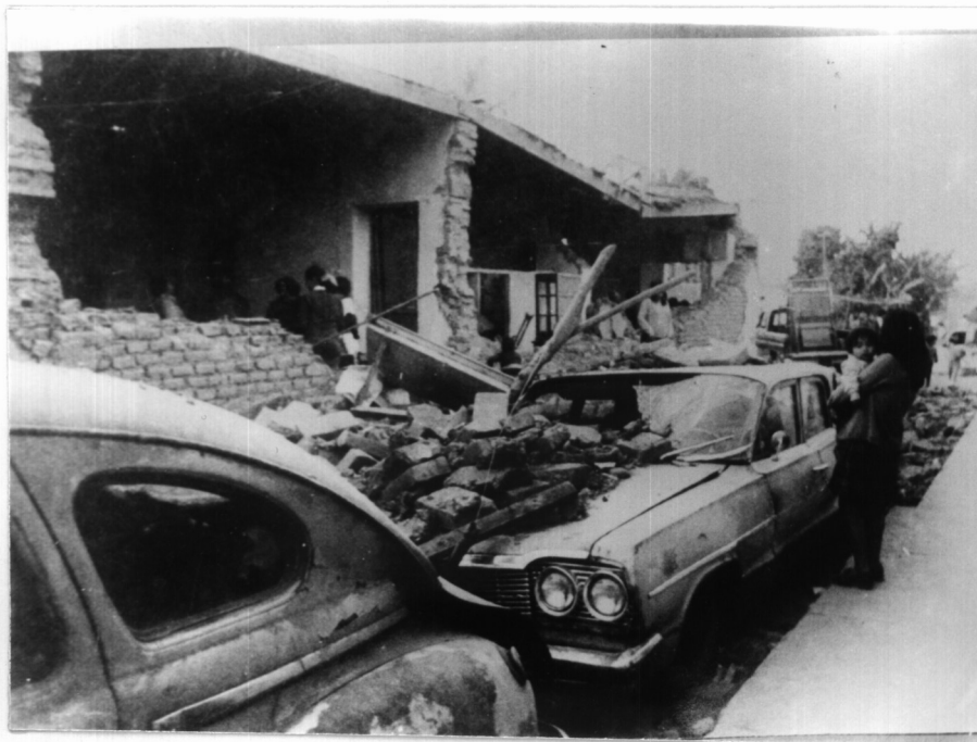
Fig. 7 Collapse of Adobe Houses in Ancash, Peru, after the May 31, 1970 earthquake.
