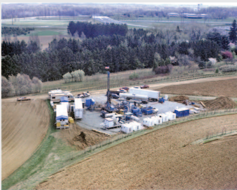
FIGURE 5.1 Drilling in the Newark Basin, New Jersey, using an offset drilling method.
