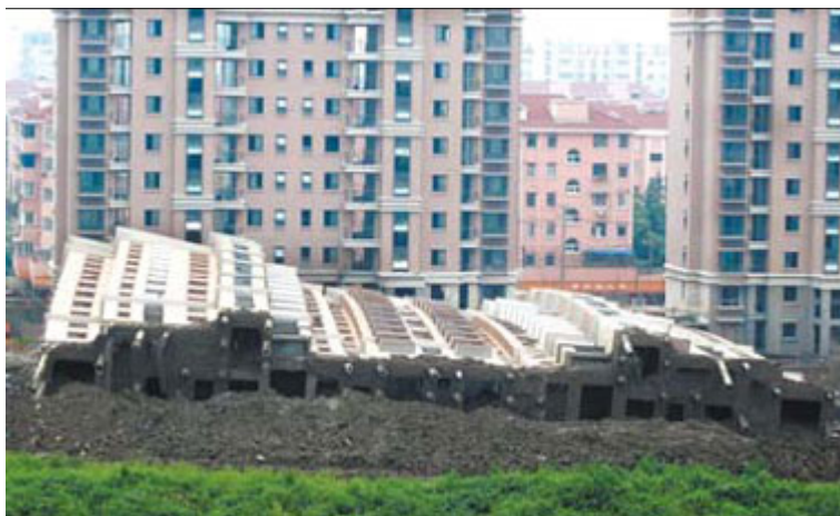
The 13-story apartment building, which was under construction, toppled over almost intact, killing one worker. Gao Erqiang
