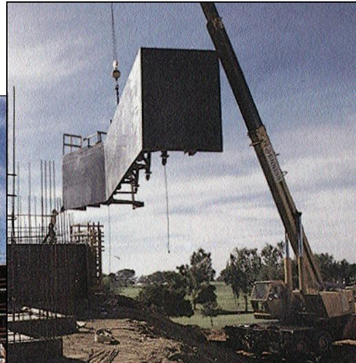
Half tunnel form, enough for walls and deck of half a hotel room, lifted by crane to its position on one wing of the 400-room hotel (left). Closer view (above) shows the 30° bend designed into each room module.
