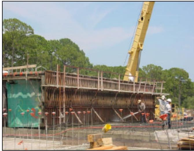
Propane heaters may be placed in the bays between wall forms to accelerate curing and the open ends of the bays are covered with canvas. After curing over night at 120 to 150 degrees F, the 3,000-psi concrete (the typical concrete used) reaches strength of 1,600 to 1,800 psi, strong enough so that the forms can be stripped.
