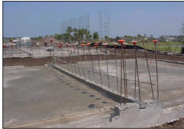
After the starter wall forms have been stripped, room-length sheets of welded wire mesh are tied to the rebar. The rebar provides continuity of reinforcement for each floor level from the floor below. Tunnel forms are then placed by crane between the rows of reinforcement, butted against the starter walls for alignment, and leveled with the screw jacks. Electrical conduit is installed and box-outs for doors, windows, and other openings are placed in precut openings in the wire mesh.
