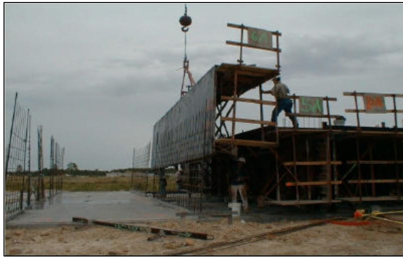
Forms for the other side of each wall (which may also be tunnel forms) are then placed. Spacers are used to center the wire mesh between the forms. The inclined struts that are an integral part of the tunnel form are adjusted to insure that the ceiling panel is positioned at the proper height. The struts transfer the load of the concrete to the base of
