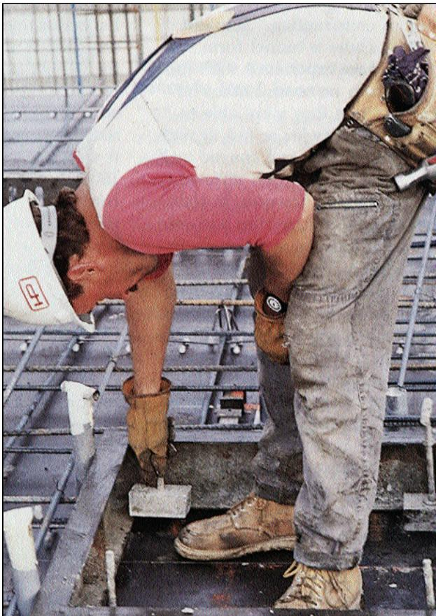
Worker places permanent magnets that attach small blockouts to the steel deck forms. The magnets are strong enough to hold the blockout form in place during concreting, and they eliminate drilling holes in the deck.
