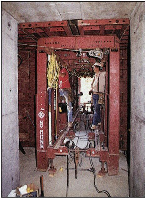
A modified box culvert form was used to make hallways, with integral slab-and-wall tunnel forms set on either side. The culvert form was moved lengthwise down the hall from pour to pour.
