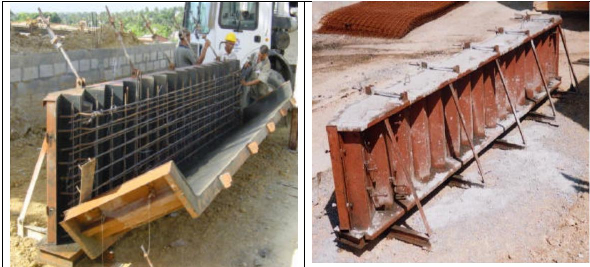
The forms, plus the heated curing, allow concrete to be placed on a daily repetitive basis. Cost, Quality, and Precision Building dimensions are reportedly held to within 1/32 of an inch. This level of precision allows plumbing elements and electrical conduit to be precut to size, leaving only installation to be done in the field. A key element in achieving this level of precision is the starter walls that serve as the guide for aligning the tunnel forms.
