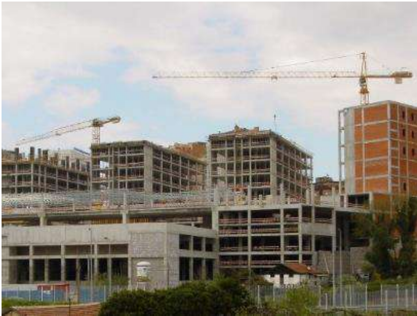
Bare Frame RC structure – Stage 1
