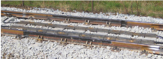
Figure 13 — Rail expansion joint (REJ) in ballasted track
