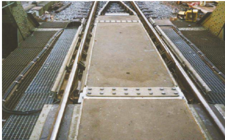
Figure 14 — Rail expansion joint (REJ) in embedded rail
